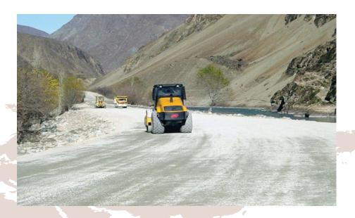
general, a single lane of the road is 3.75 meters. The road will consist of the following sections:
