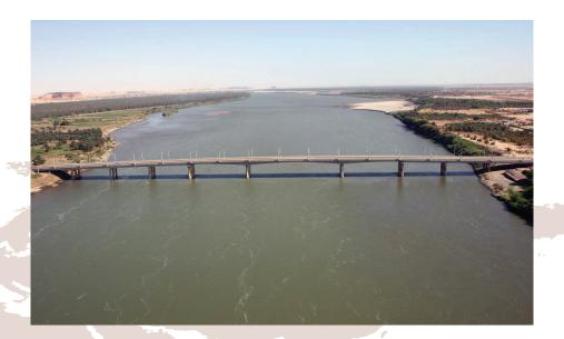
long and 9.60 meters wide with two lanes, each 3.65 meters wide and two pedestrian platforms each 90 cm wide.
