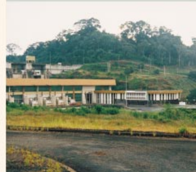
Song Loulou Hydro-Electric Power - Cameroon
