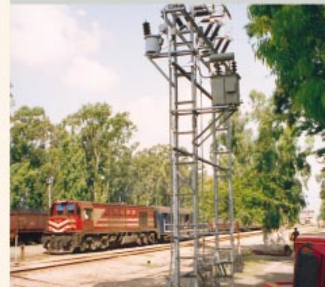
Modernization & Electrification of Iskenderun - Divrigi Railway Line - Turkey
