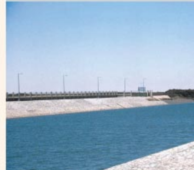
Irrigation Canal for Sina Dessert - Egypt
